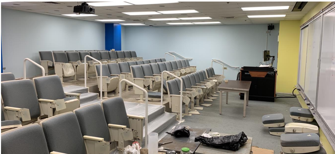
POST 723, part-way through its renovation and painting.
